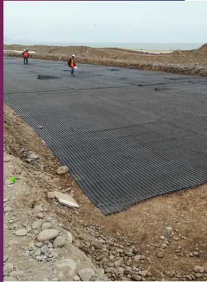
Dynamic loads and constant trafficking have a direct impact on railway infrastructure. Preserving track alignment and preventing ballast displacement are keys for optimized performance. The use of Geoquest geogrids will reduce ballast settlement and degradation under the influence of traffic, will reduce maintenance and increase service life, therefore resulting in long term savings.
